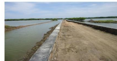
Talud Penahan Jalan
