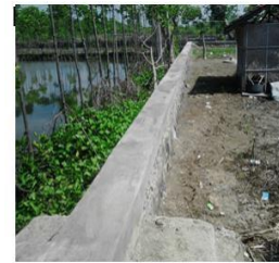
Talud Penahan Rob
